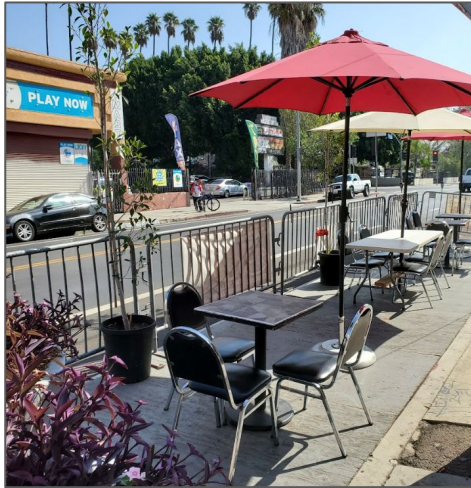
No Structural Review: Wood deck and freestanding barriers and umbrellas
