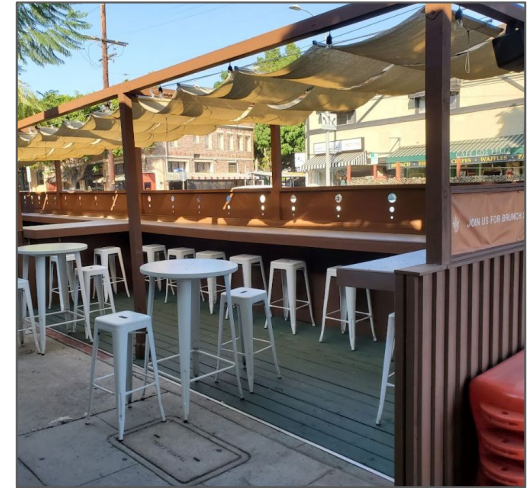
Structural Review: Structure with vertical posts and roof
